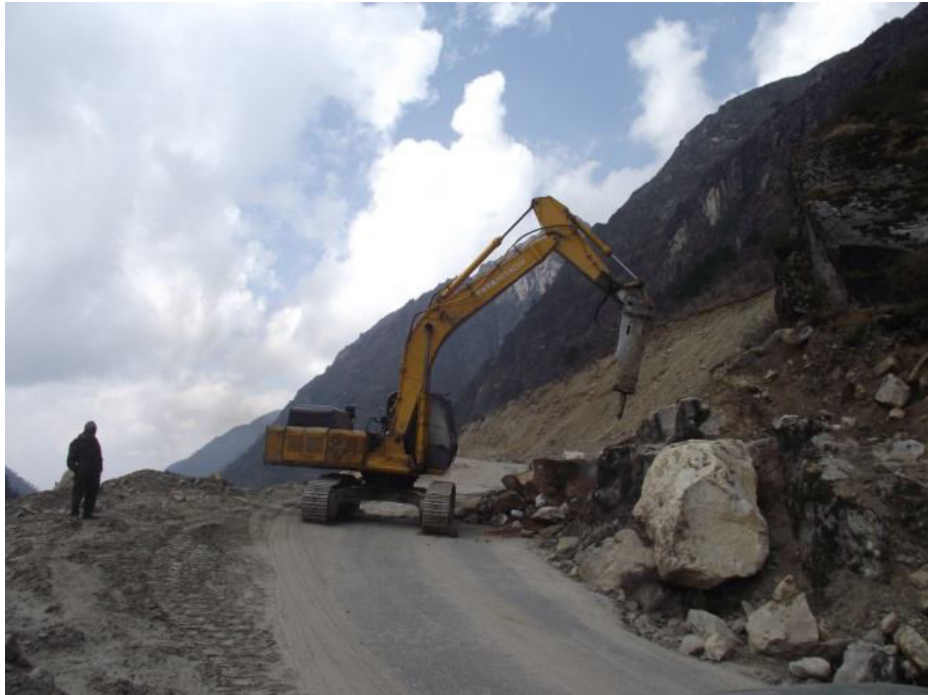
Picture 5 Slope Excavation for Widening of Road bench in Debris material
