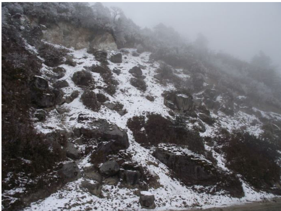
Picture 2 Debris slide with formation of Cone at the base of the Slope
